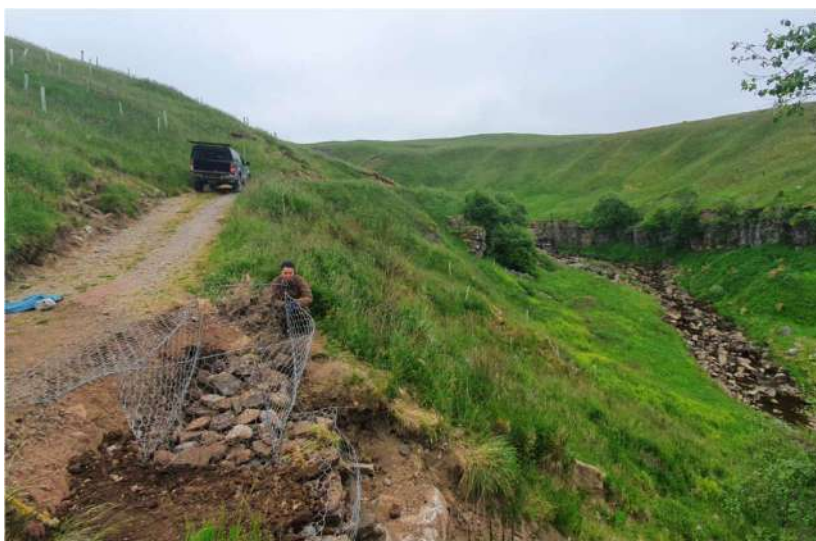
Constructing gabion baskets
