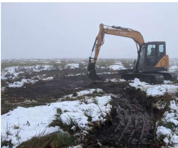
Phase 1 wetland work ~ creating wader scrapes
